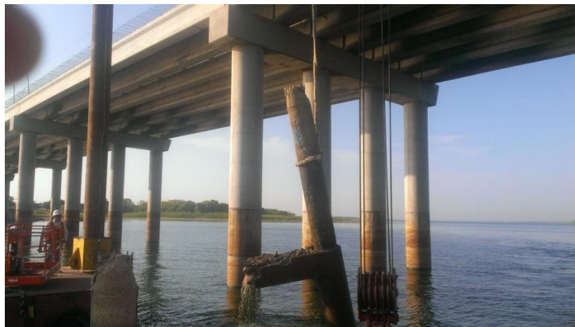
Positioning the Shearer for Tie Beam Cuts
