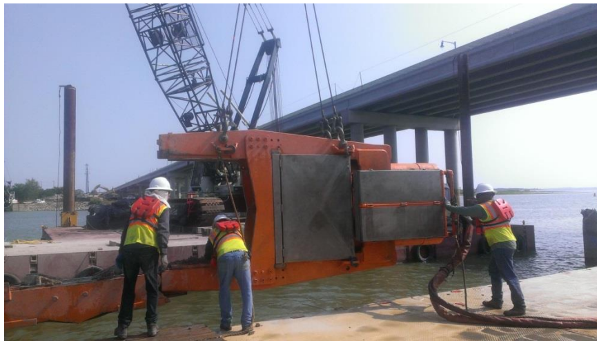
Positioning the Shearer for Tie Beam Cuts
