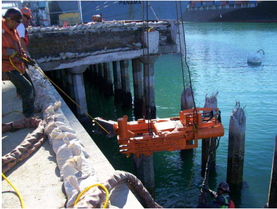
Lowering the shear into position for each cut takes just minutes.
